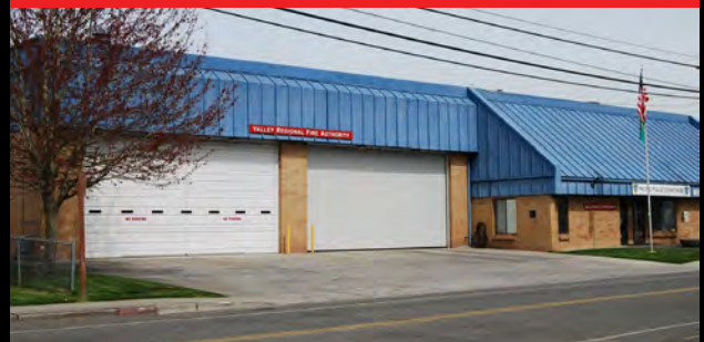
STATION 38 | PACIFIC 133 3RD AVENUE S.E., PACIFIC, WA
